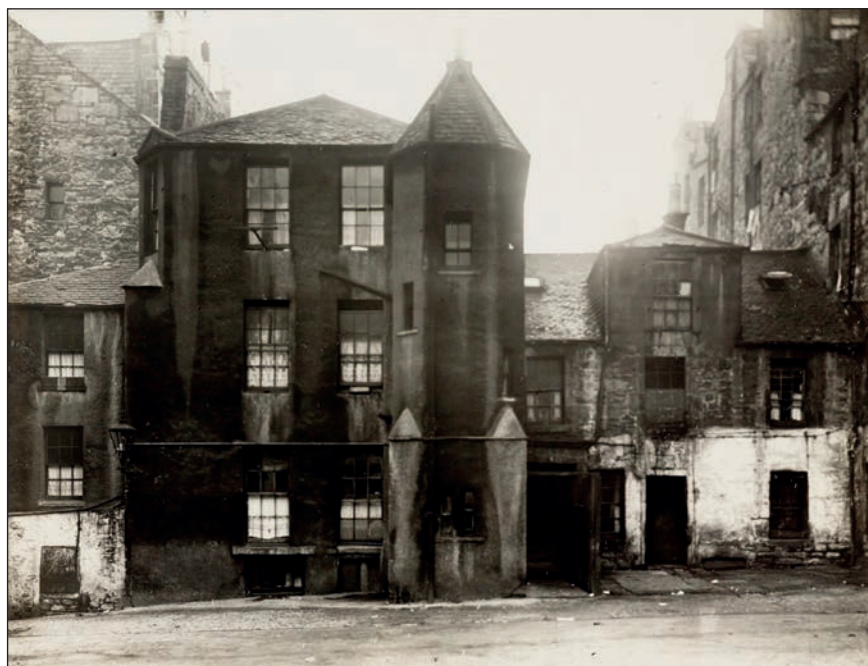
Fig. 1. The building housing the first Synagogue in Scotland in Richmond Court, taken in 1929 by Alfred Henry Rushbrook. Reproduced with permission of the National Library of Scotland
